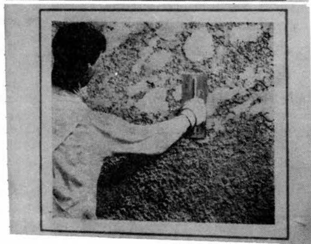
Two steps in the Italian Travertine finish, from 1920s stucco finishing handbook.
